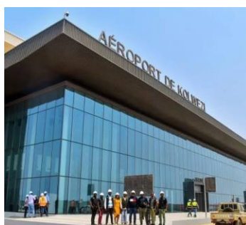
New Kolwezi Terminal
