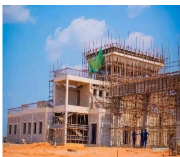
Control Tower-Mbuji Mayi
