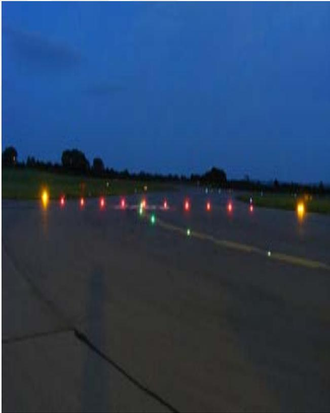
A series of unidirectional red lights, embedded in the pavement, right angles to the taxiway centerline, at the associated runway holding position, the lights are spaced 3 meters apart ,across the taxiway located 0.3 meters before the holding point lines.
