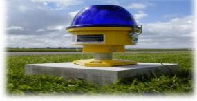
Delethalisation. Below ground ramping to buried vertical face of construction designed to reduce risk of damage to aircraft running on cleared and graded area of strip.
