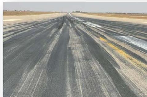
Beginning of destruction of the internal tire 600 m from the threshold
