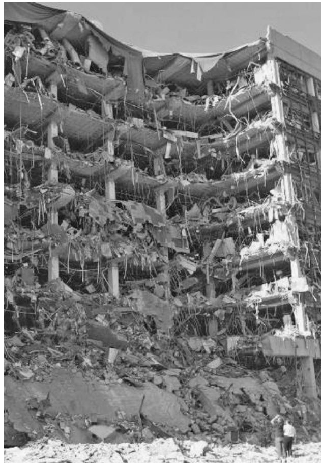
Progressive collapse witnessed in the aftermath of the Oklahoma City bombing in 1995
