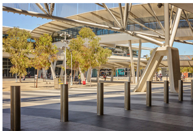
Impact rated bollards – Courtesy of Adelaide Airport
