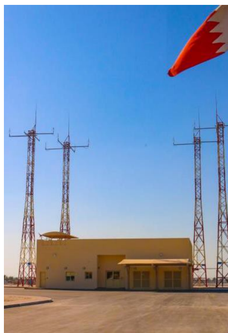
Figure 1. New Transmitter Station
