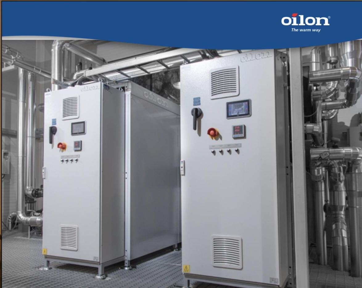
In May 2016, two Oilon P380 heat pumps (Finland) were installed to extract heat from the Duty Free Shop to pump it into the rest of the Airport. The new system completely eliminates the use of fossil fuels for heating and is 400% more efficient than the boilers.
