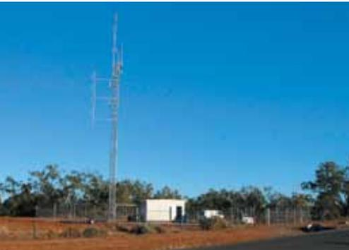
cial air traffic in Australia is currently under radar coverage, over 90% of Australian airspace is outside radar coverage. The Automatic Dependant Surveillance Broadcast (ADS-B) system has provided extensive coverage in non-radar airspace and complements the existing en-route and terminal radar RASPP network
