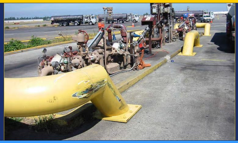
This loading station is protected against physical damage by ground vehicles.
