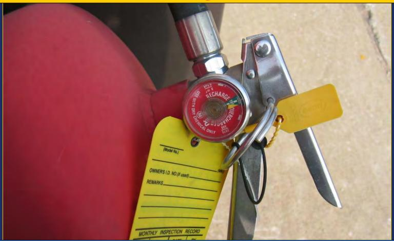
Check fire extinguishers for proper charge, pin sealed and current inspection tags. Extinguishers should be inspected at least annually by a fire extinguisher servicing company.
