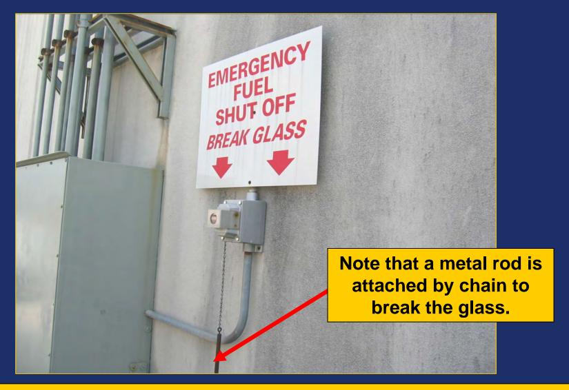
NFPA 407, 4.4.5.7 (continued) Any action necessary to gain access to the shutoff device (e.g., BREAK GLASS) shall be shown clearly.
