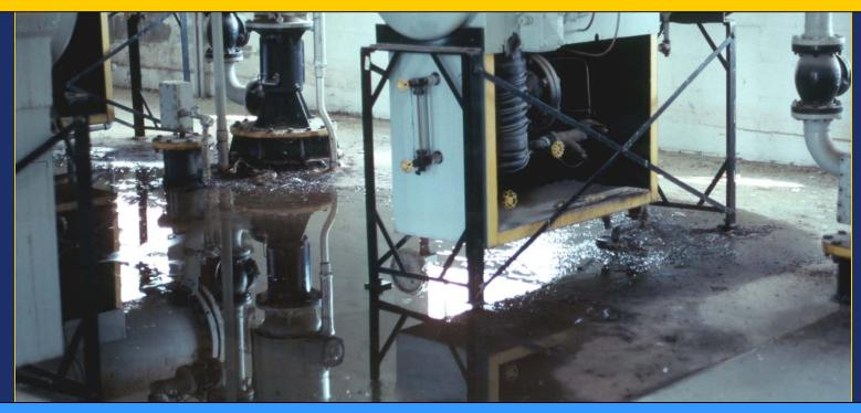
This fuel servicing equipment is leaking and is not being maintained in safe operating condition.
