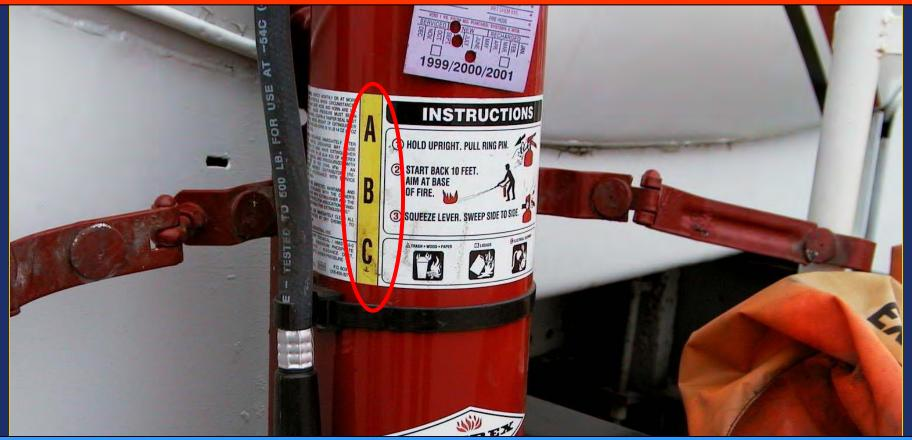
Dry chemical extinguishers are the most common type used. Dry chemical extinguishers must be B C rated. ABC rated multipurpose dry chemical extinguishers are highly corrosive to aircraft and can cause significant damage to aircraft engines.
