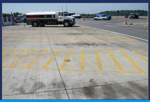
Marking the parking locations for fuel trucks to ensure compliance with parking standards is highly recommended. Note that the oil stains indicate fueling personnel are complying with the parking standard.
