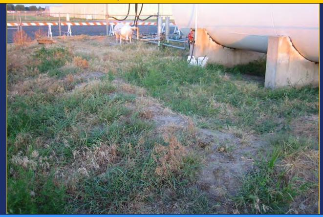
The ground area around this tank storage facility is not free of weeds, which can contribute to the spread of fire.
