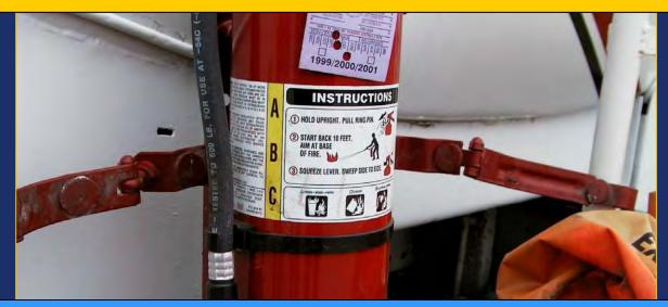
When fueling agents have their fire extinguishers inspected, extinguishers from hangars sometimes get mixed up with extinguishers from fuelers. This dry chemical extinguisher needs to be replaced with a B C rated dry chemical extinguisher.
