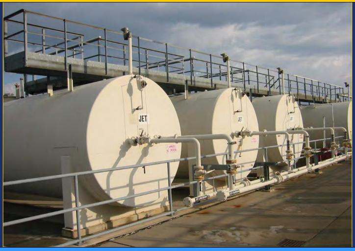
Above ground fuel tanks need to be grounded or bonded together and connected to a grounding rod.
