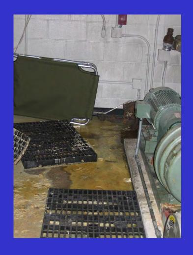
These reserve foam tanks leaking at their piping joints, creating a mess and walking hazard in the rapid refill storage room.
