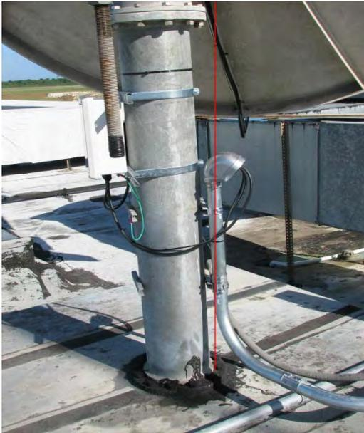
Elevation jack screw upper pivot is elongated – causing 4 degrees of movement
