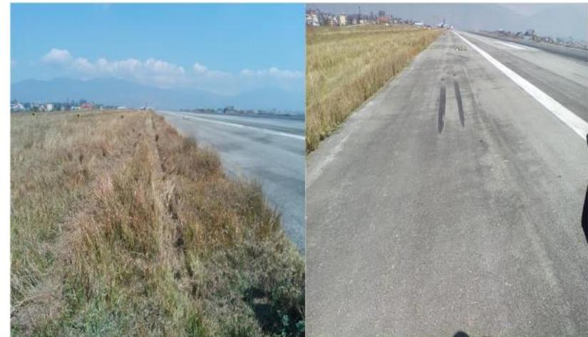
Initial touchdown points of Left and Nose landing Gears
