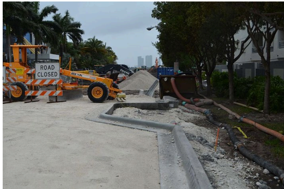
Raising roads and increasing drainage capacity in Miami-FL
