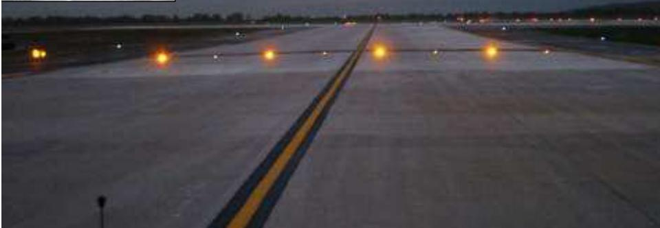
Elevated and In-pavement Runway Guard Lights are a common RSAT recommendation to enhance the identification of runway-holding positions at intersections with a history of runway incursions.
