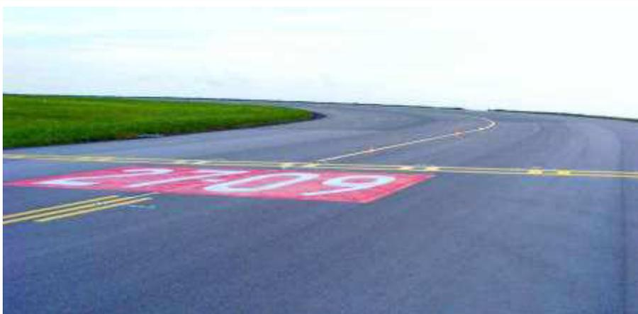
**ENHANCED RUNWAY DESIGNATOR MARKING AT PATTERN B HOLDING POINT**
