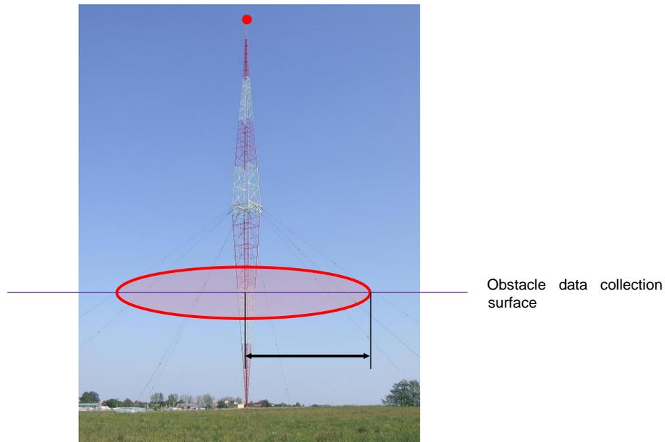
Figure A3: Capture of the relevant elevation and extent of a mast with guy wires
