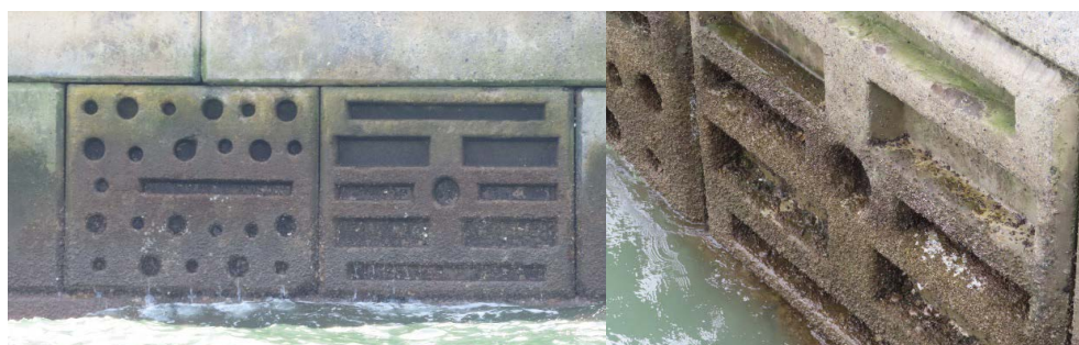
FIGURE 2: Eco-enhanced vertical seawall blocks
