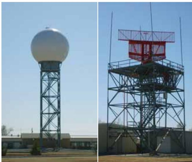
**TDWR (left) experienced early problems with outages that have now been resolved. The ASR-9 system, right, has been upgraded with implementation of WSP. Less costly than TDWR, WSP allows for wind shear prediction at medium-capacity airports; however, it does not perform effectively in a dry environment**
