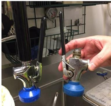
During the summer of 2018, the Airport Authority offered free water assessments to all food and beverage tenants, followed by free low-flow pre-rinse spray valve replacements and aerator installations. As part of the program, 49 pre-rinse spray valves were replaced and 96 aerators installed, resulting in an estimated 16,862 m<sup>3</sup> of water savings per year (Figure 5).
