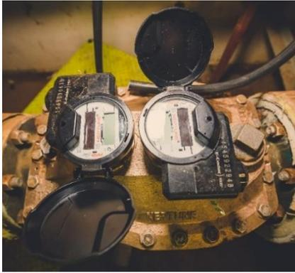
Water metering is necessary for managing water use more effectively by detecting leaks and improving the accuracy of unaccounted and unmetered usage. In 2017, the Airport Authority installed new water meters in all terminal buildings (Figure 2). The Airport Authority has also improved water metering of its irrigation system.
